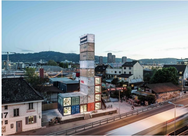
10: FREITAG store in Zurich by spillmannechsle, 2006
