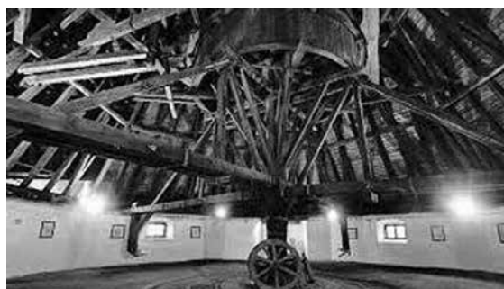
Gápel nad šachtou Leopold, NKP Solivar
